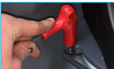
Mount the Smartseat Easy Tip Fold on single seatleg with 4 bolts M10 x 35 quality 10.9 or higher. Tighten these bolts to 50 Nm.
